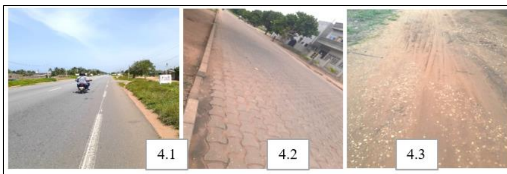
Plate 4: Road infrastructure in the Grand-Popo arrondissement
