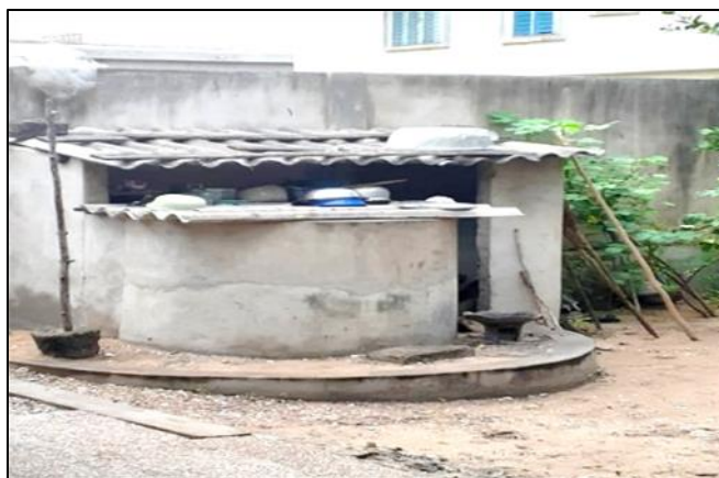
Photo 1: Well in some households in the Grand-Popo arrondissement
